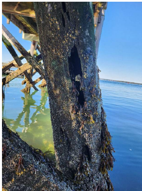
Photo No. 12: Pile with severe checking, splitting, and section loss.
